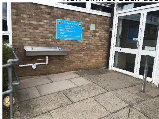
New sink at back door
